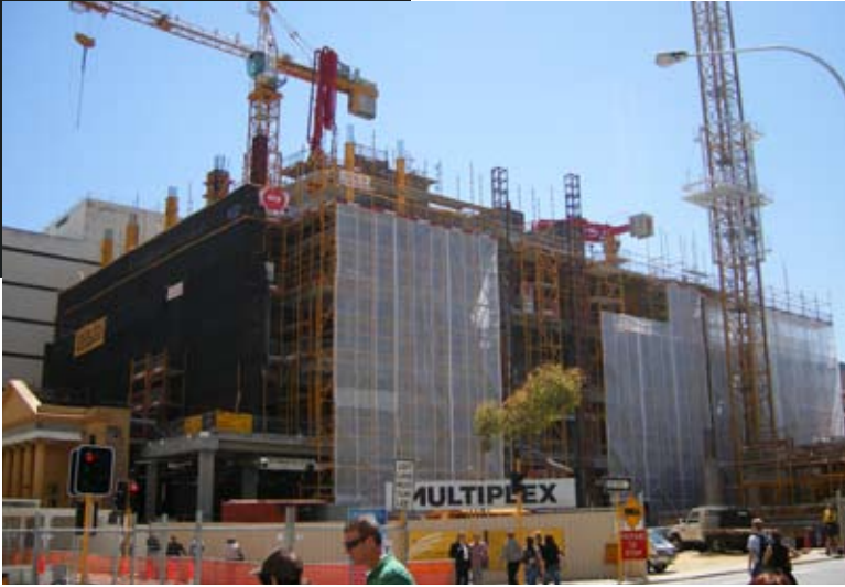
Construction underway with heritage facade incorporated (at left)
