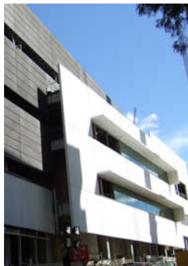
Feature precast concrete facade
