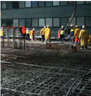
top: Pre-existing footings are uncovered
