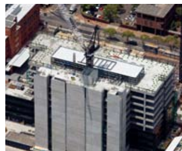
White precast concrete western facade walls on the Justice Administration building
