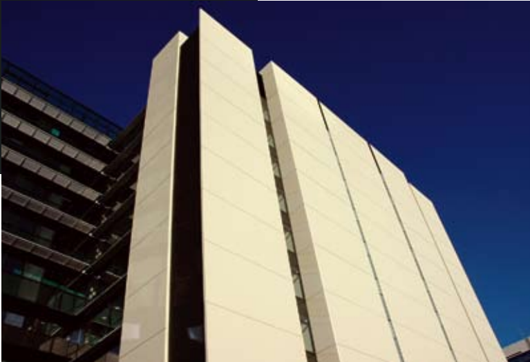
The all concrete Justice Administration building achieved a 5-star Green Star rating
