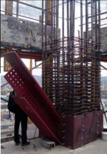
Integration of the 'mega' steel braces required unique connection detailing
