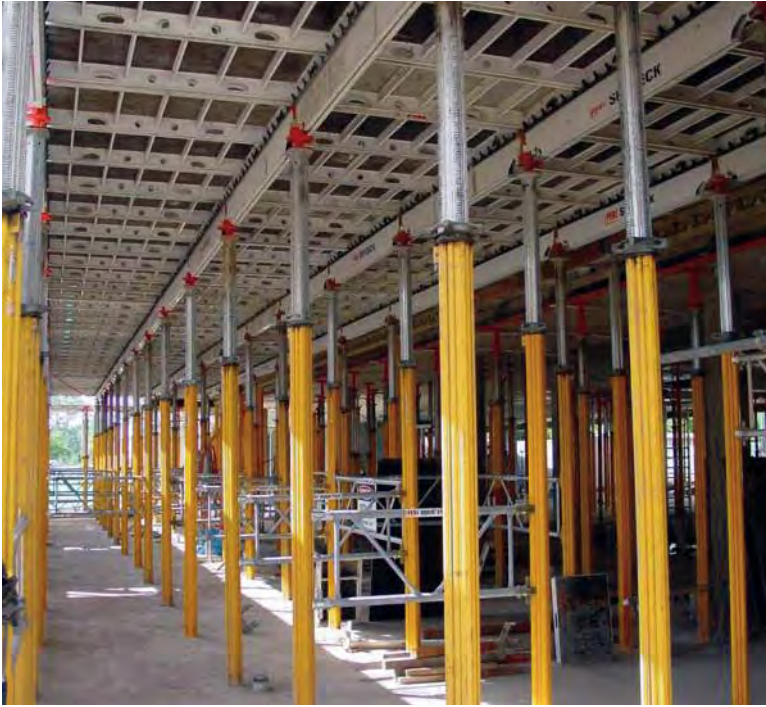
Figure 3 The 'skydeck' modular system by PERI is an example of the newer generation of floor form systems
