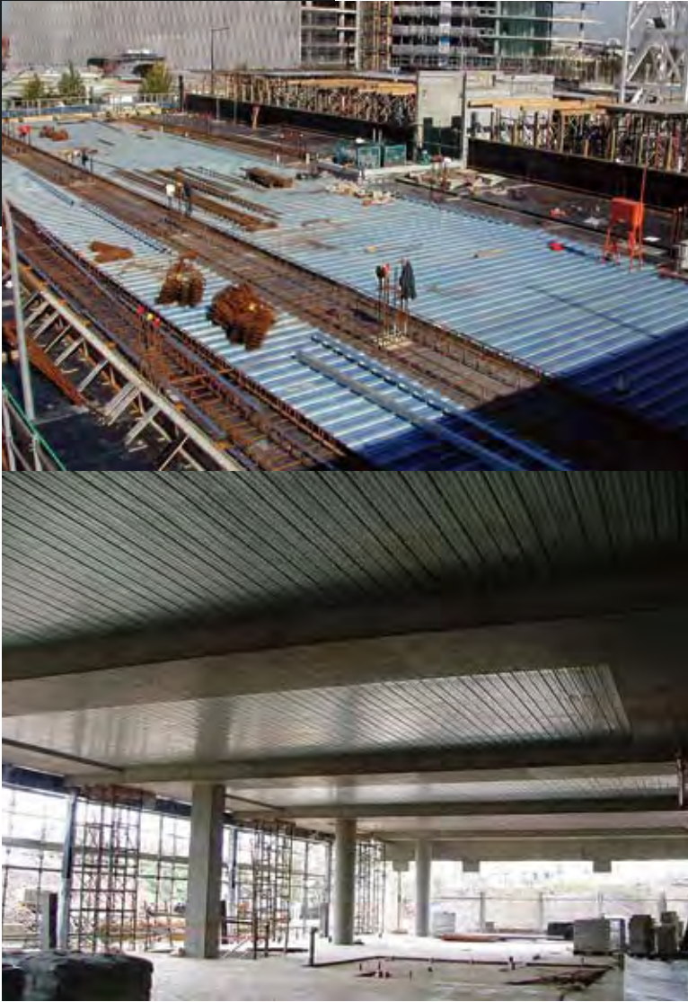
Figure 4 Permanent metal deck formwork
