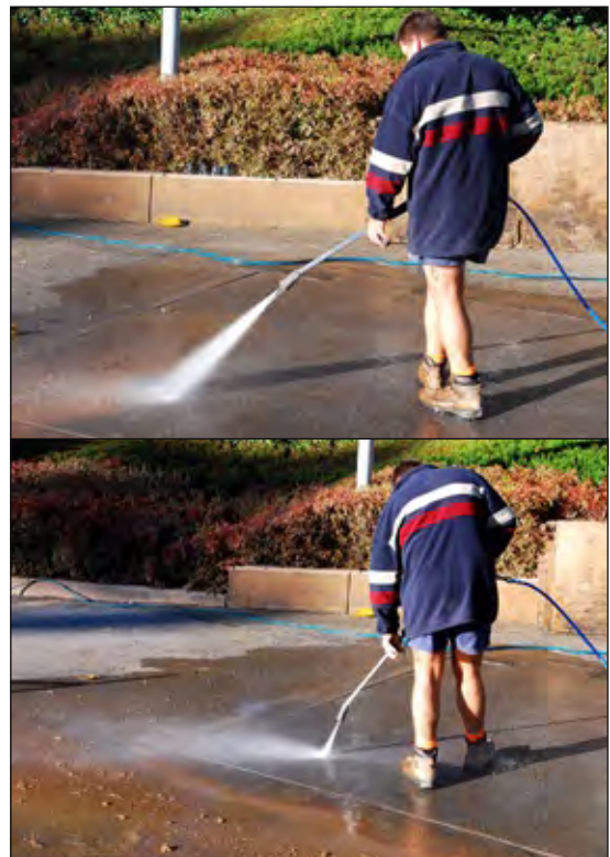
Figure 2: Pressure washing pavement – nozzle distance adjusted depending on force required to dislodge dirt
