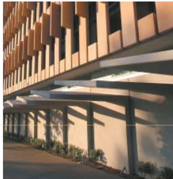
6 Precast awning components
