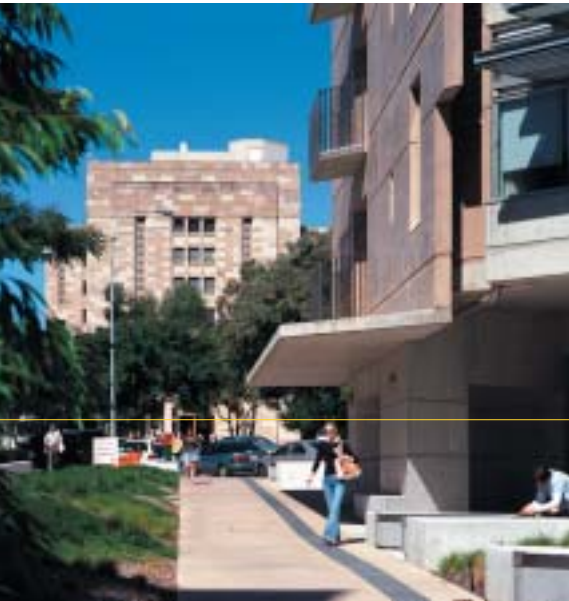
2 View of the Forgan Smith Building from GPN3
