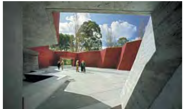
Four coats of red dye sprayed onto walls to achieve deep yet translucent red colour. (Shrine of Remembrance Courtyards, Melbourne)
