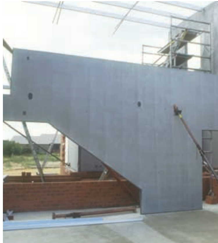
Concrete Panels allow architectural design freedom and loads such as floors and stairs to be supported.
